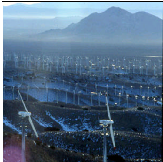
The Tehachapi Pass area in Central California has the potential to greatly expand its wind power resources but requires substantial improvements to the transmission system to deliver the energy. Photo by Sean Ramsay, courtesy of The Energy Overseer .
