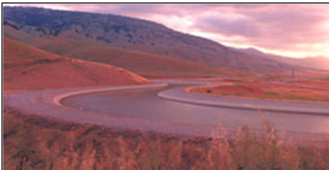
The 444-mile long California aqueduct carries massive amounts of water to farms and communities in Southern California. Photo courtesy of DWR.
