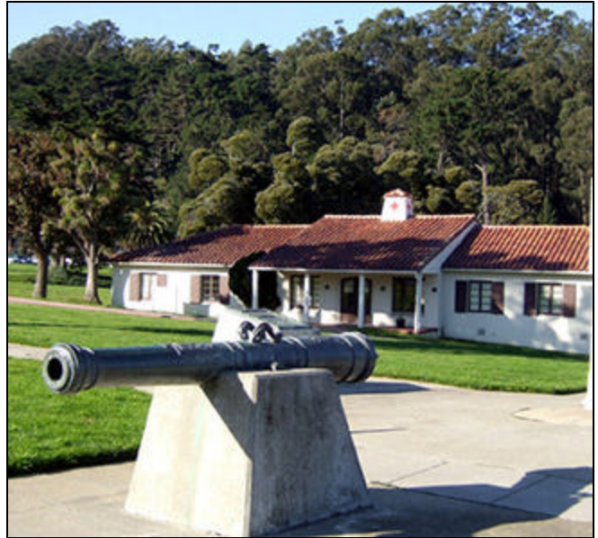
This building, a former Army base clinic now occupied by the nonprofit Center for Resource Solutions, would be demolished for construction of the CAMP proposal, but could be preserved under the Presidio Historical Association's proposed museum plan. Photo by Arthur O'Donnell.
